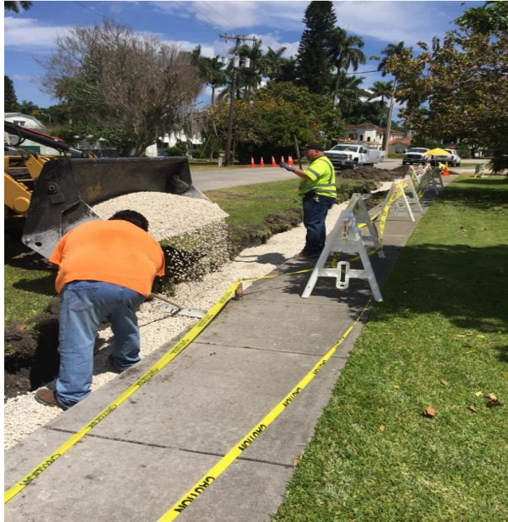
Street Crew installing a French Drain on Arcade
